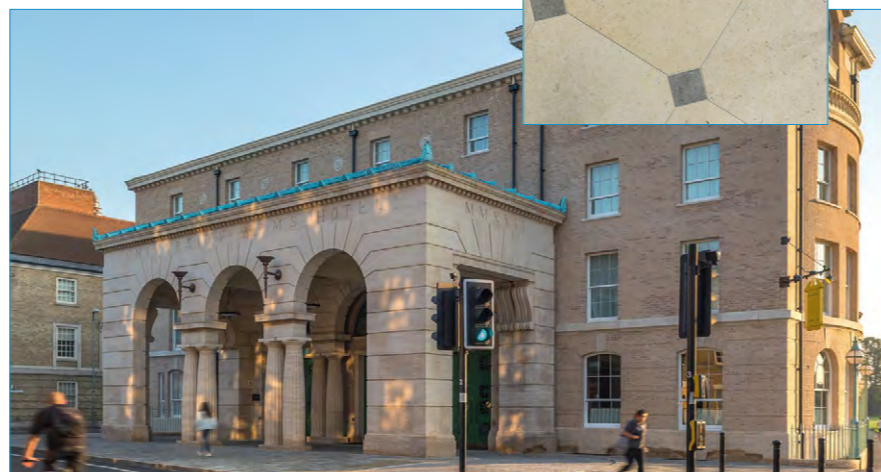
Stamford Stone (F56) supplies its own Clipsham and Lincolnshire limestone and imported stone for a wide range of projects.
