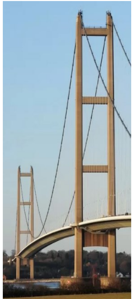
The Humber Bridge, the gateway to Hull. Opened in 1981 by HM Queen Elizabeth II. It held the world record for the longest single span until 1998.
